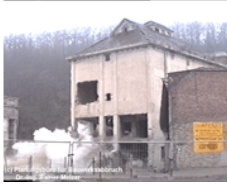
Figure 1: Reference structure in Weida/ Germany
